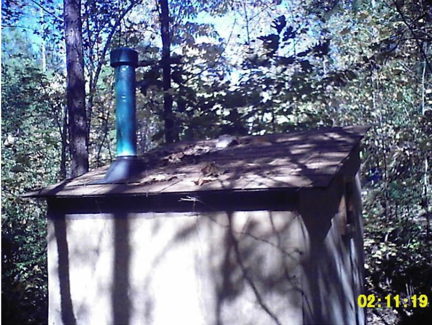
I shingled my roof in the standard manner. Note the vent pipe made of 4" PVC. An oversized cap is on top to keep water out. Holes were drilled in the end of the pipe to allow extra ventilation. Screen was wrapped around the pipe to keep the bugs out.
