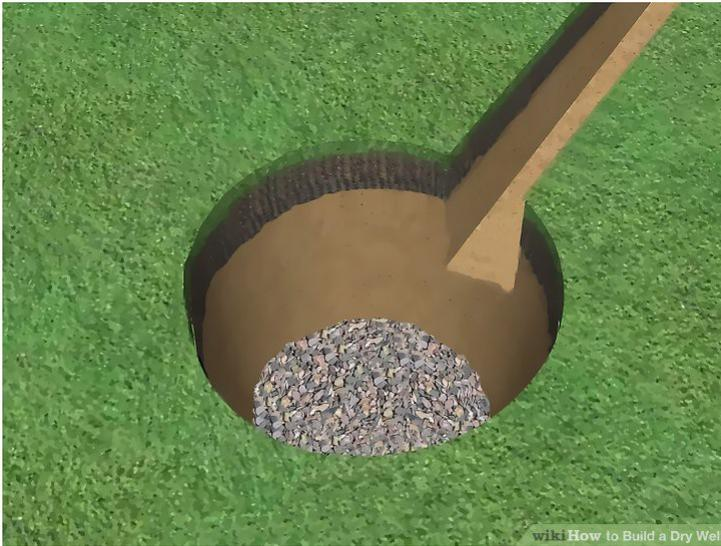
3. Spread approximately 2 inches (5 cm) of gravel along the bottom of the trench and bottom of the holding tank pit.
