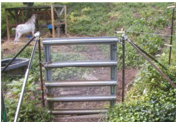
This is the gate to our buck area. It is hung using the special hardware they make for t-posts. It has worked fairly well and I would recommend it for use with does or wethers, but if we did this again, for bucks, we would probably sink wooden posts. The bucks used to stand on, and stick their head through, the gate, but Larry covered it with hardware cloth, which has now made it impossible to stand on and so the gate is holding up much better.
