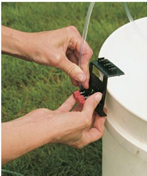
2. Attach tubing to each of the three ports on the gang valve. Plug bubblers into the other ends.
