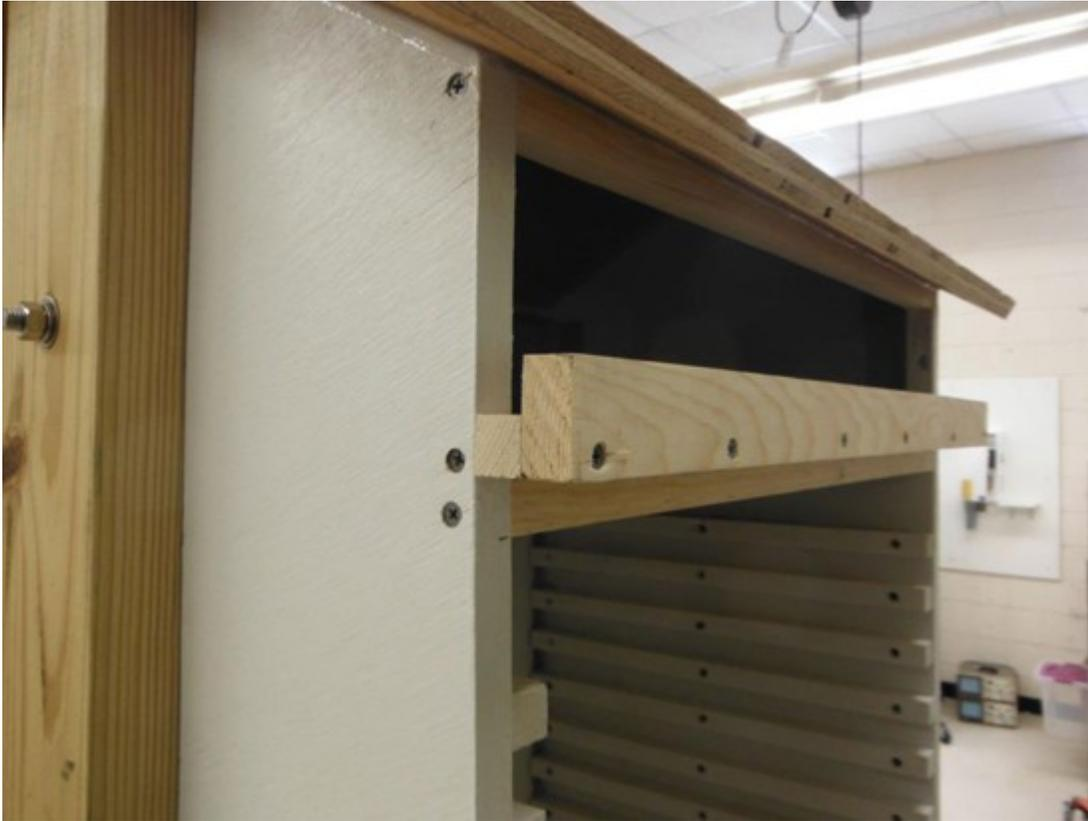
To install the back vent covers, you'll first need to build up the 1-1/2-inch-wide brace at this location so it can support both the covers and the door (which you'll install next). Attach a 3/4-by-3/4-by-24-inch strip of wood to the top half of the brace, and then screw a 1-1/2-by-3/4-by-24-inch wooden piece to the top of the strip you just placed on the brace. Drill pilot holes to avoid cracking the wood, and be sure to stagger the screws for the first and second strips.
